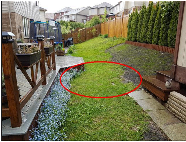
4.4 SITE GRADING Image 1
