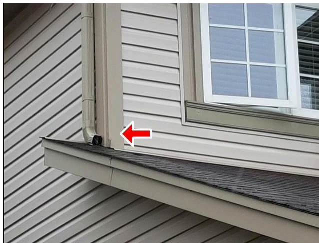
1.5(1) DOWNSPOUTS / ROOF DRAINS Image 1
