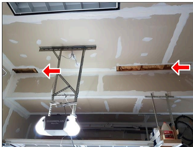
5.1 WALLS / CEILINGS Image 1
