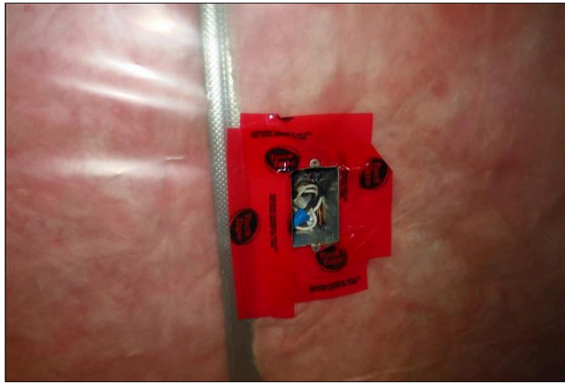
12.3 WIRING / CONDUCTORS (EXPOSED) Image 1
