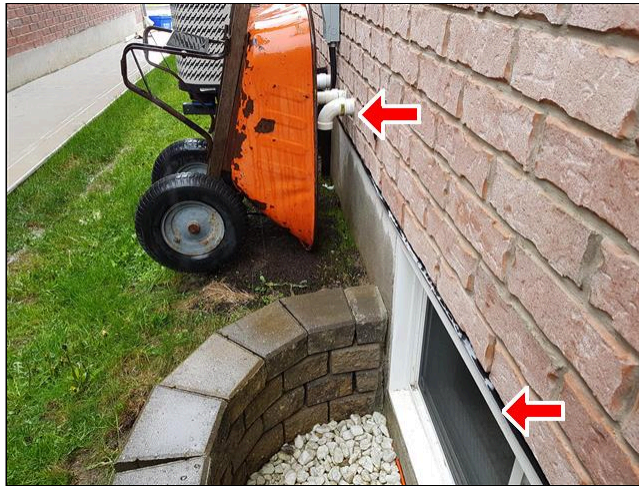
3.11 DRYER/OTHER EXTERIOR VENTS Image 1
